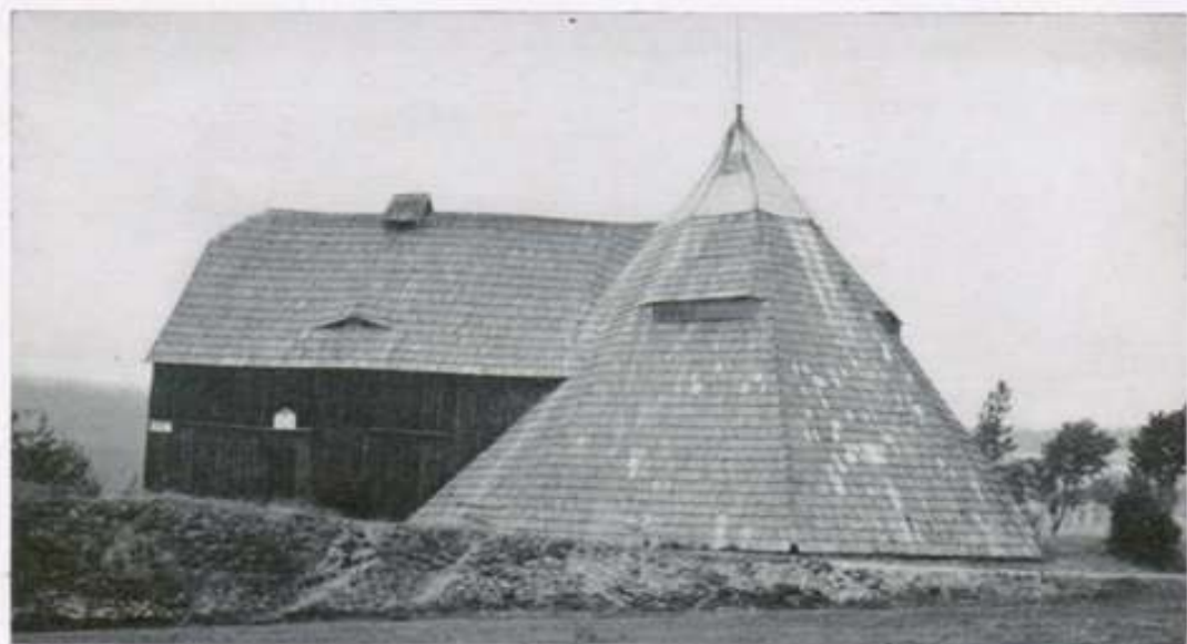
(Below) The Pferdegöpel at Johannegeorgenstadt. The last survivor of horse-powered mine shafts, over 200 years old
